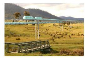
Unlike road or rail systems, because the system is elevated it can traverse mountains or other rough terrain and is not constrained by earthworks, embankments, sleepers and ballast, with minimal environmental impact at ground level.
