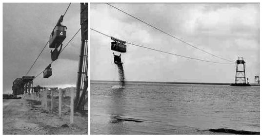
For example, the system of the company Neyrpic (France), which was established in the framework of the project "Delta" for the construction of the dam foundation "Grevelingendam" between the islands of Schouwen-Duiveland and Goeree-Overflakkee in 1963–1965.
